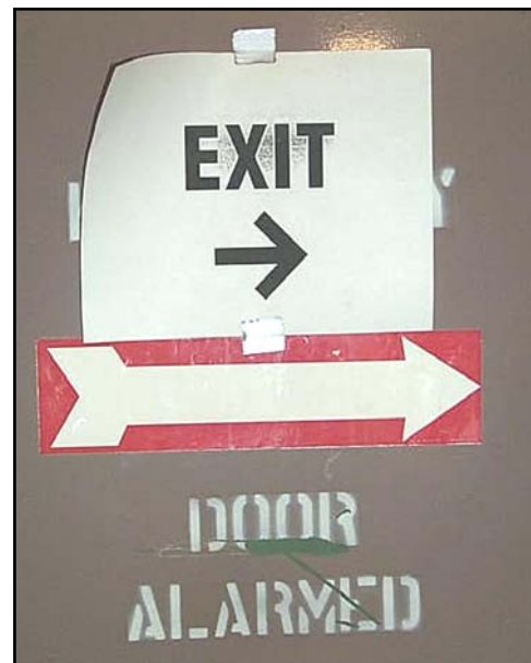
Figure 2: Improper paper Exit sign
