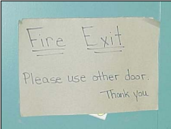
Figure 1: Improper handwritten Exit sign
