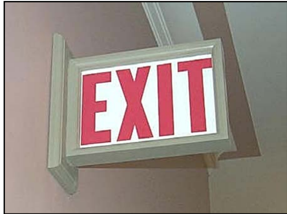
Figure 4: Exit sign illuminated by an adjacent light
