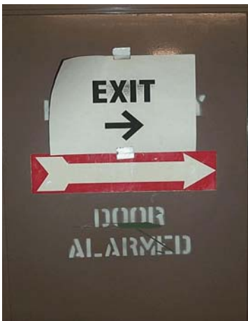
Figure 1: Improper paper Exit sign
