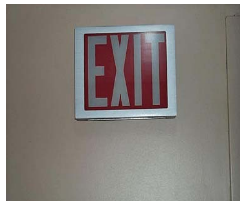
Figure 2: An externally illuminated Exit sign
