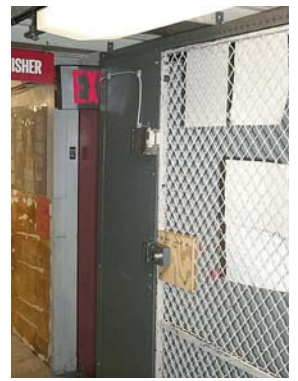
Figure 3: Blocked Exit sign
